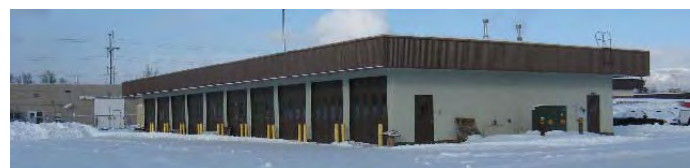
Figure 5 – Adjacent to existing lab (in background) is this 7,500 sf – road sign shop and warehouse for signs, paint and other items. A recent inspection showed little activity around it, no tire tracks in the snow and no vehicles parked in the sizable lot surrounding it.
