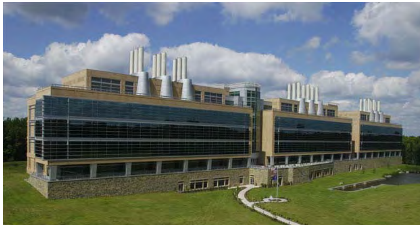
Fig. 3. FBI national headquarters. This “state of the art” crime lab in Quantico, VA opened April 2003 at a cost of $130 million to initially house 650 employees in this 436,000 sf building. [photo fbi.gov]
